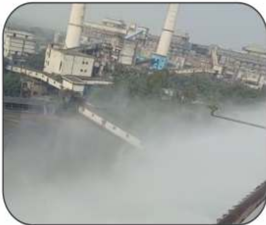
Plough Feeder Building
